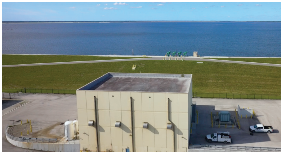
C-44 Reservoir and Stormwater Treatment Area.
