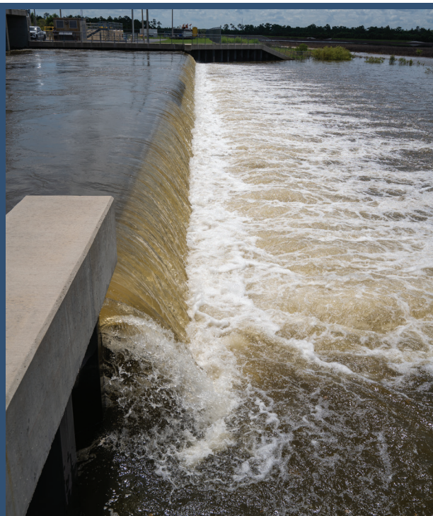
Turning on the pumps at the Picayune Strand Restoration Project.
